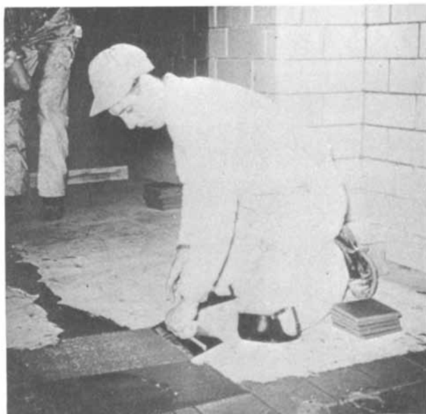
Figure 6. Spreading setting bed
