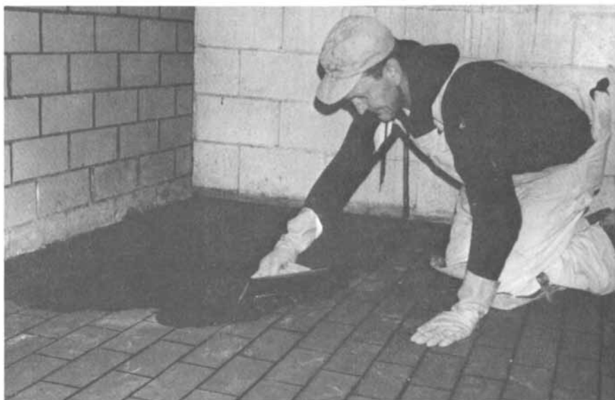
Figure 8. Grouting tile
