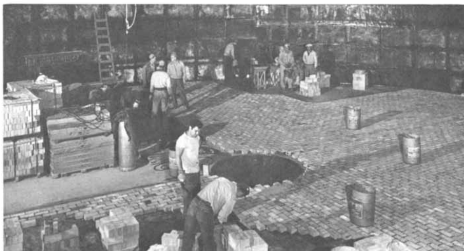
Figure 12. Installation of acid-resistant floor
