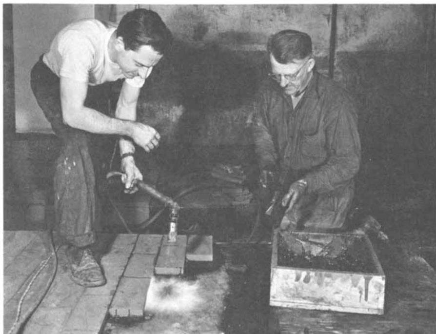
Figure 11. "Buttering" brick
