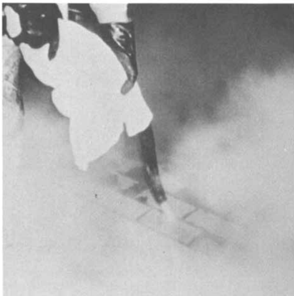
Figure 9. Steam-cleaning tile
